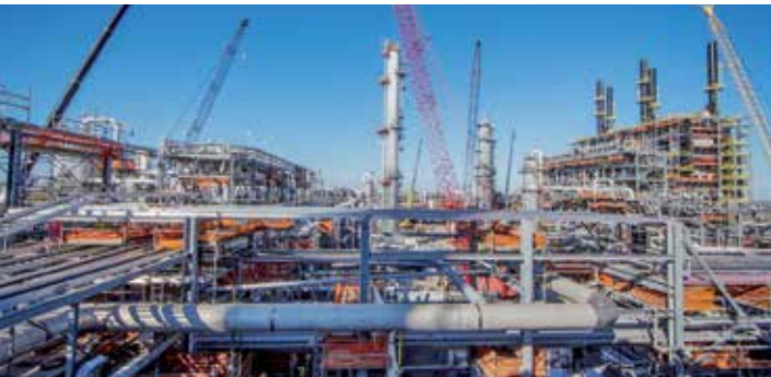
Pipeline and process plant engineering
