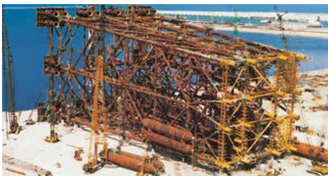
Offshore plant construction: platform
