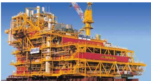
Offshore plant construction: top side
