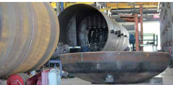
Pressure vessel construction
