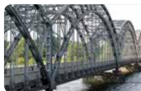
Stahlindustrie | Steel industry
